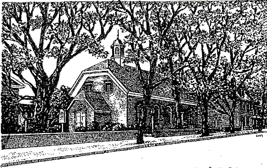
New Castle Presbyterian Church ~ Built 1707 ~ New Castle, Delaware
